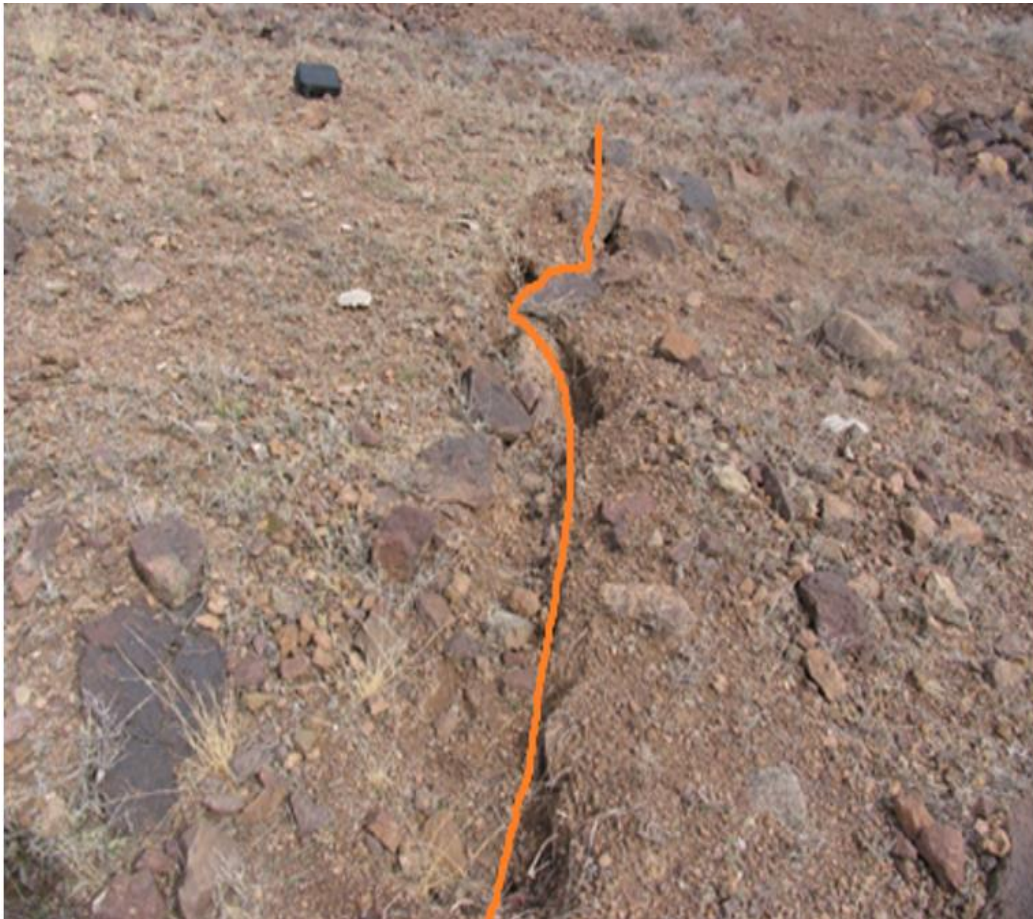
Figure 6. Second-order tensile crack.
