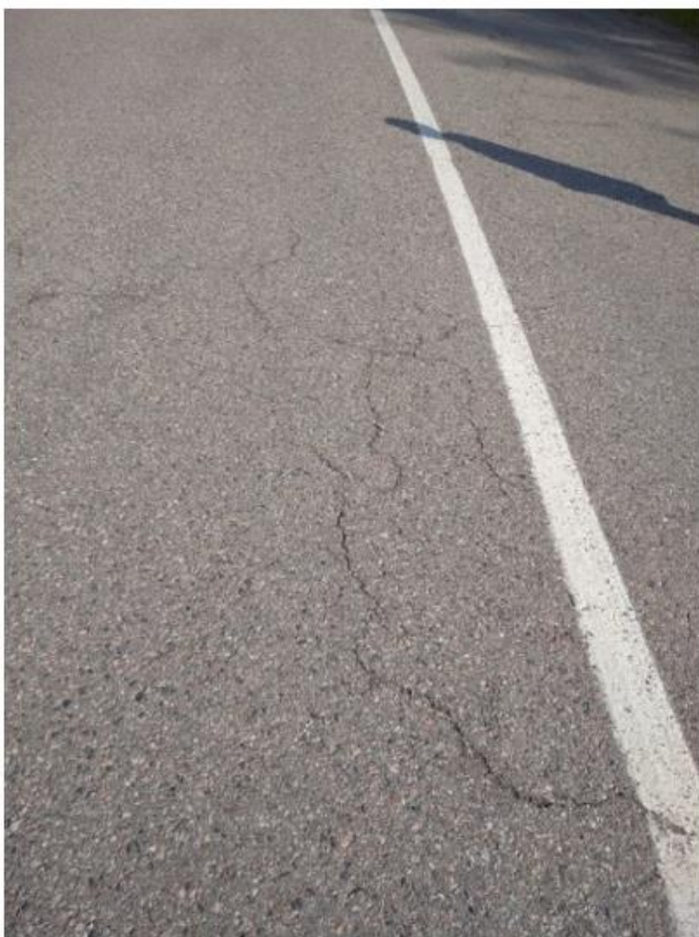
Figure 14. Small cracks and pits that appeared on the surface of the newly built site No. 5.
