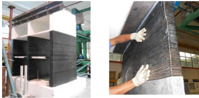
Figure-7. Wrapping of CFRP around of shear walls [44, 45].
